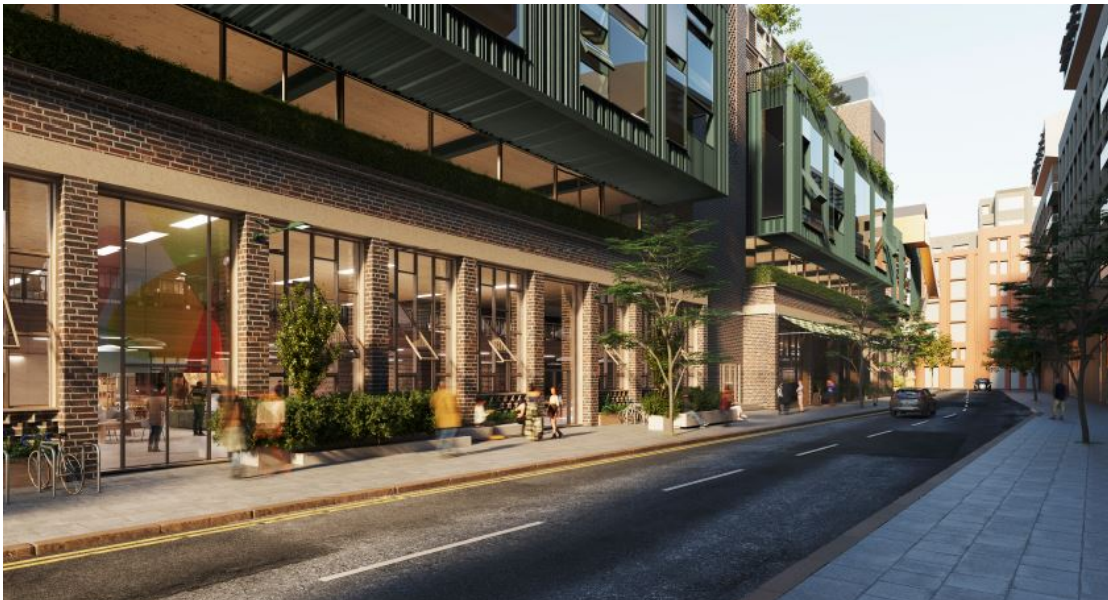
Figure 5 (above): Visualisation looking eastwards along Pocock Street. The retained brick walls of the original Court building, with sections of glazing inserted, form a 'plinth' to the new storeys above.
